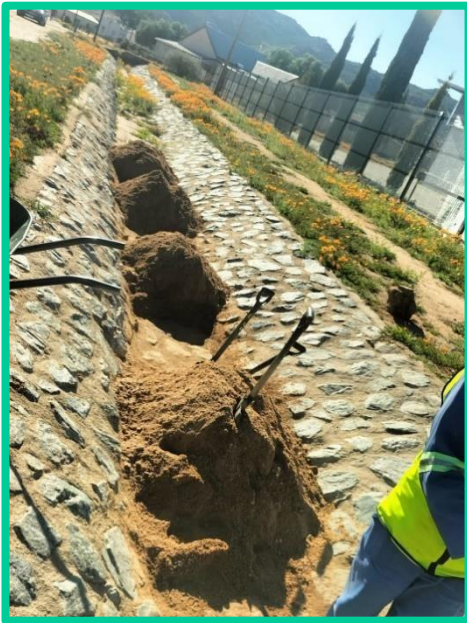
Picture 4: 800m 63mm HDEP pipe - Wheel Julia Water Network, strengthening
