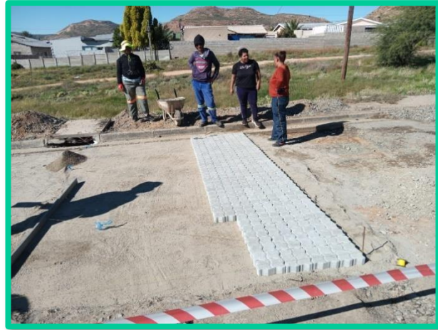
Picture 3: Upgrade of Waterkant and Skool Street intersection
