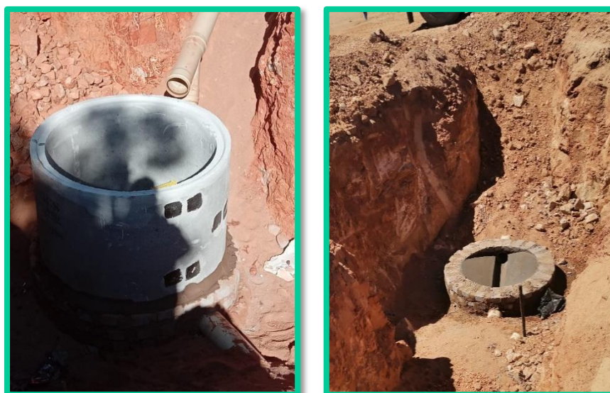
Picture 16: Okiep Sewer - Rocky Ridge project
