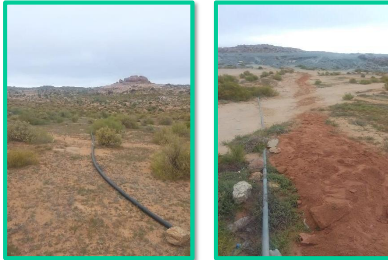
Picture 4: 800m 63mm HDEP pipe - Wheel Julia Water Network, strengthening
