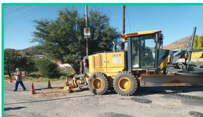
Picture 25: Upgrade of Waterkant Skool Street intersection
