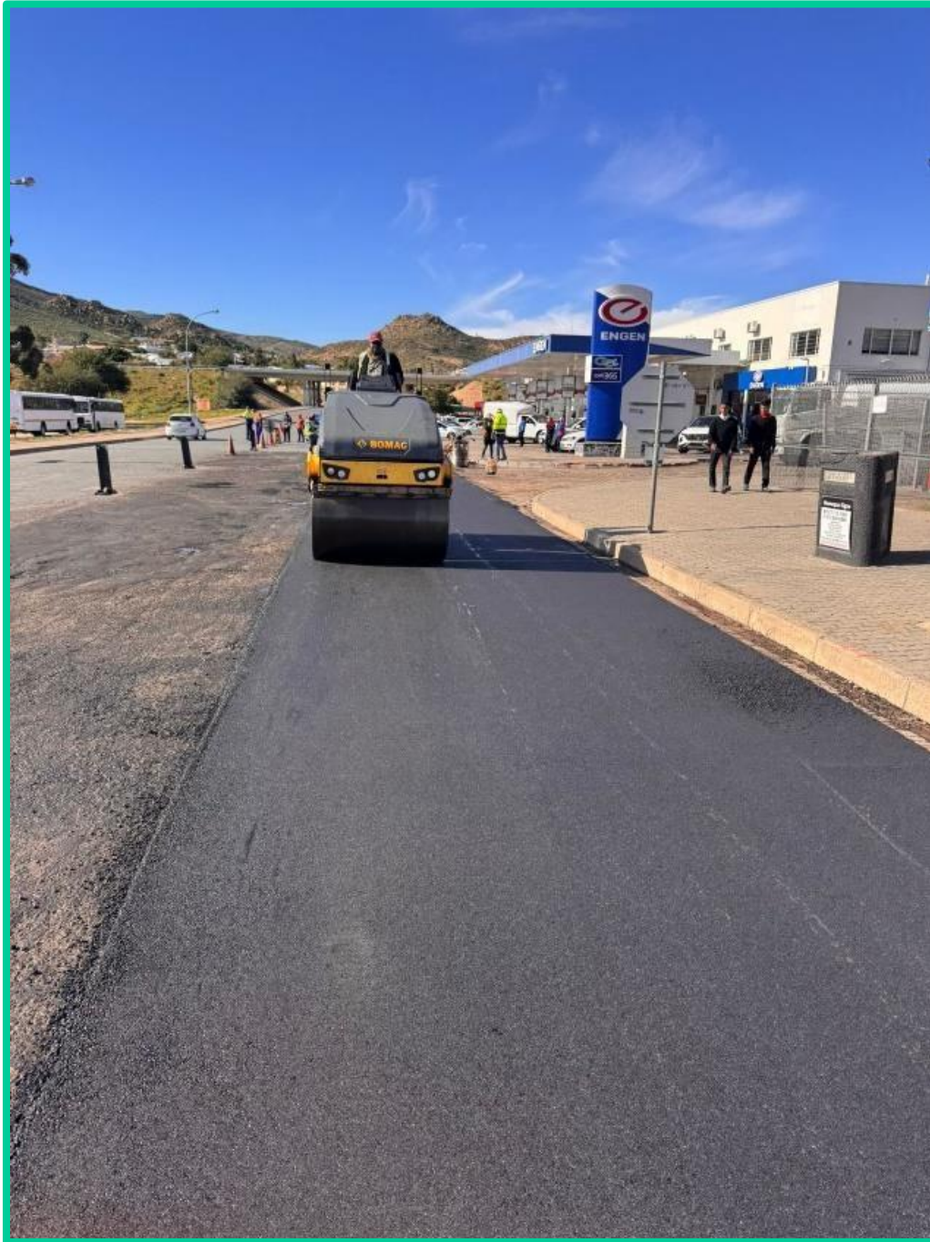
Picture 2: Slurry and tar of Voortrekker Street, Springbok CBD
