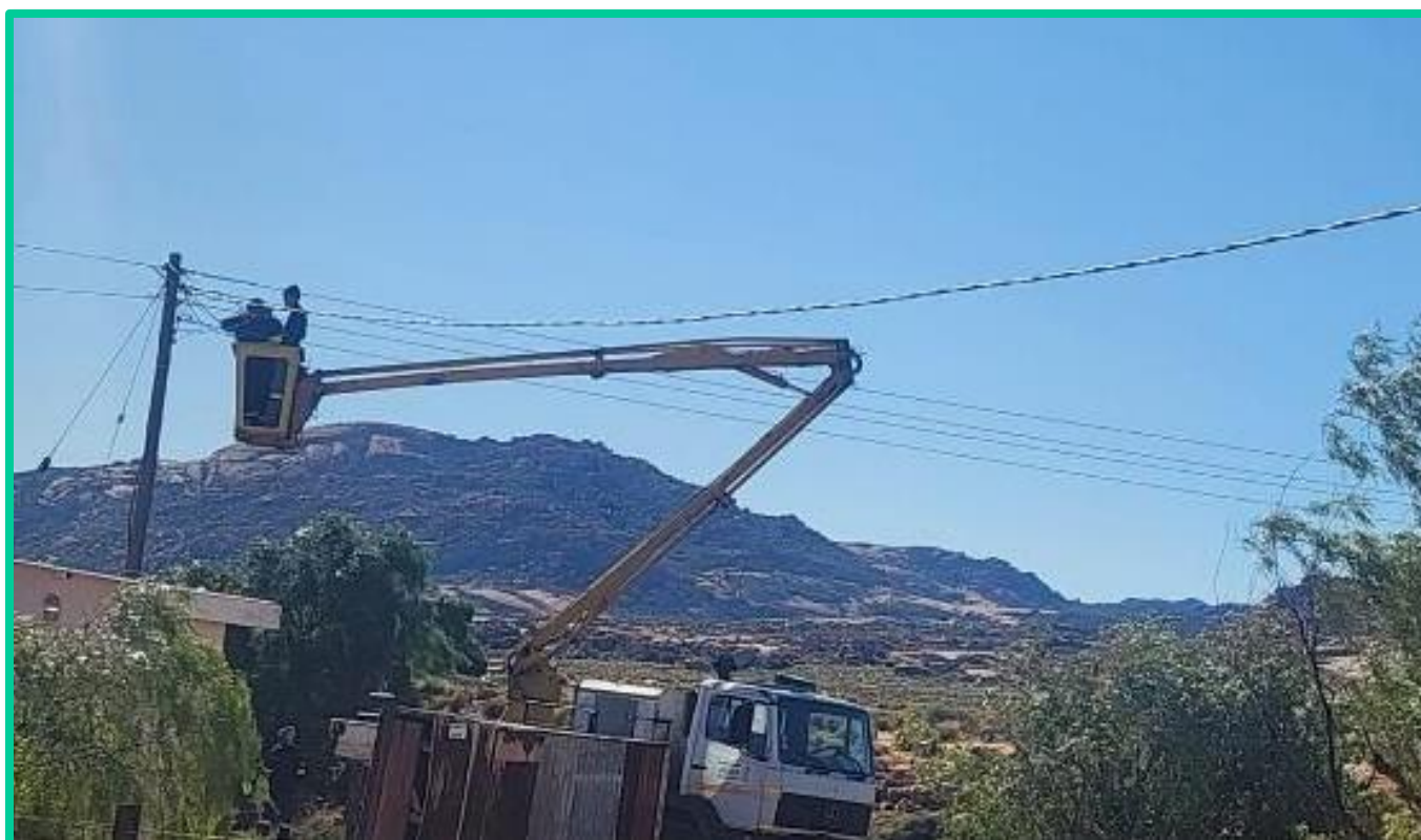
Picture 19: Routine Maintenance
