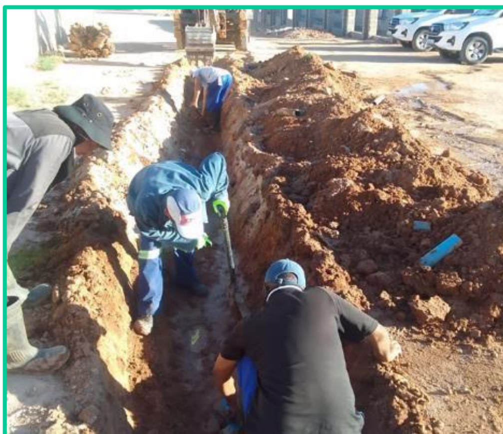
Picture 12: Routine Maintenance
