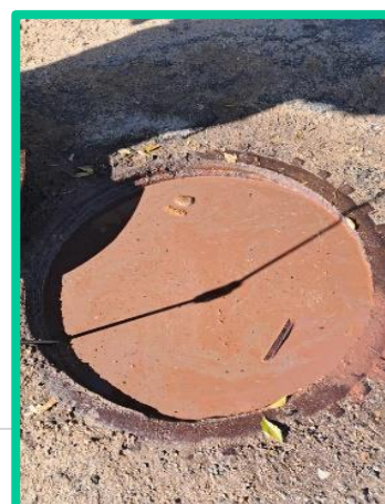
Picture 15: Routine Maintenance works
