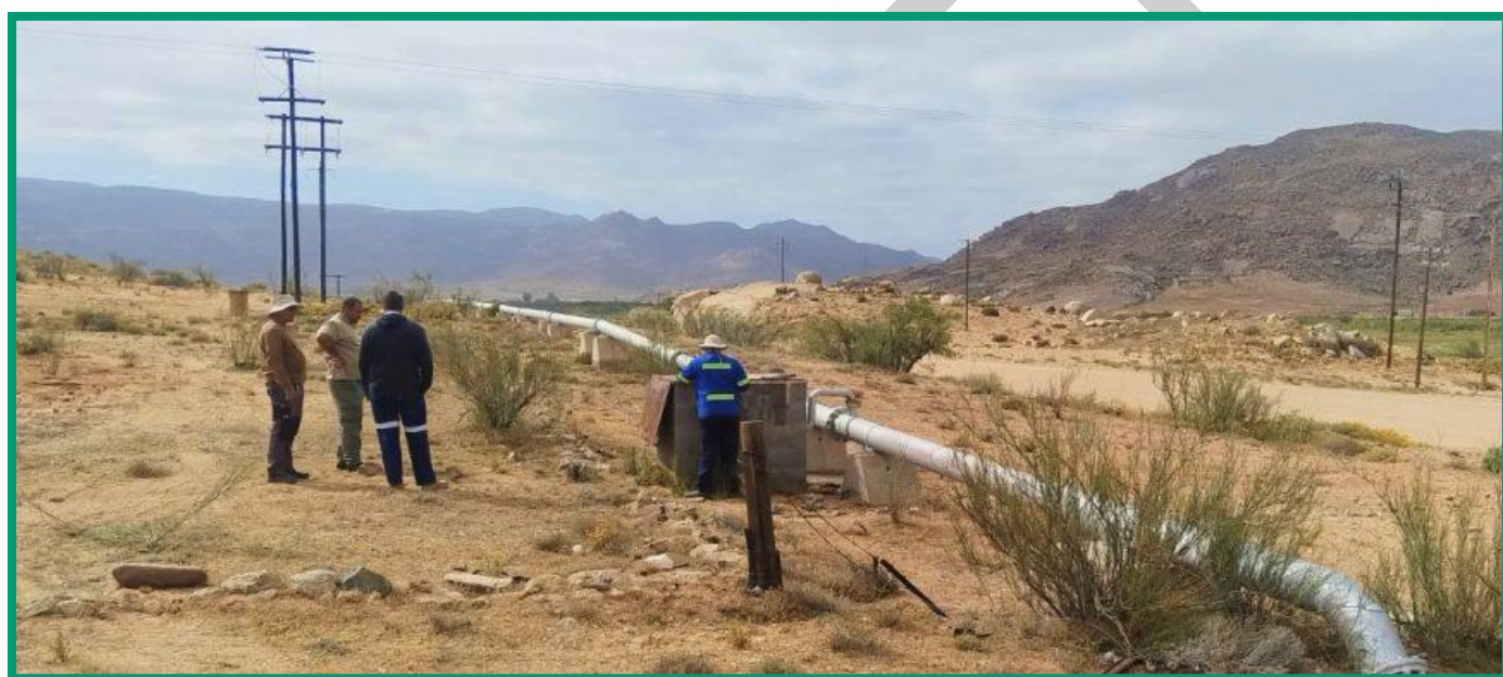
Picture 9: Upgrade of infrastructure of Buffelsrivier and Kommagas
