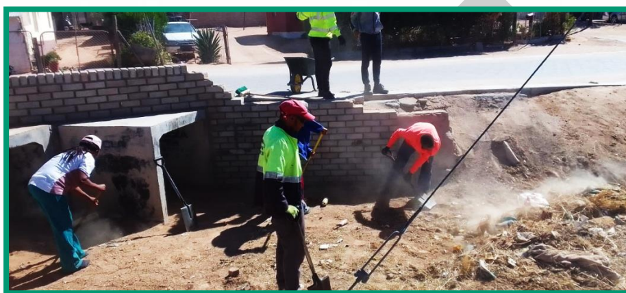
Picture 32: Clearing of stormwater channels
