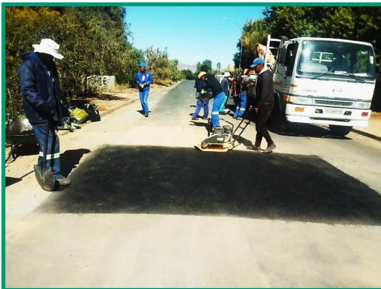
Picture 28: Municipal officials re-sealing roads and fixing potholes
