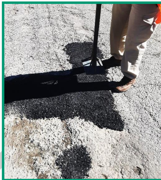
Picture 28: Municipal officials re-sealing roads and fixing potholes
