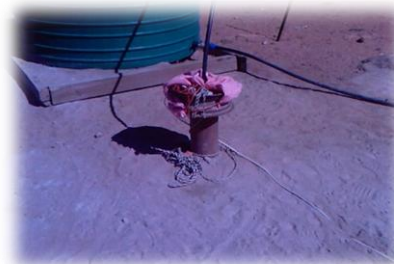
Borehole 100m depth
